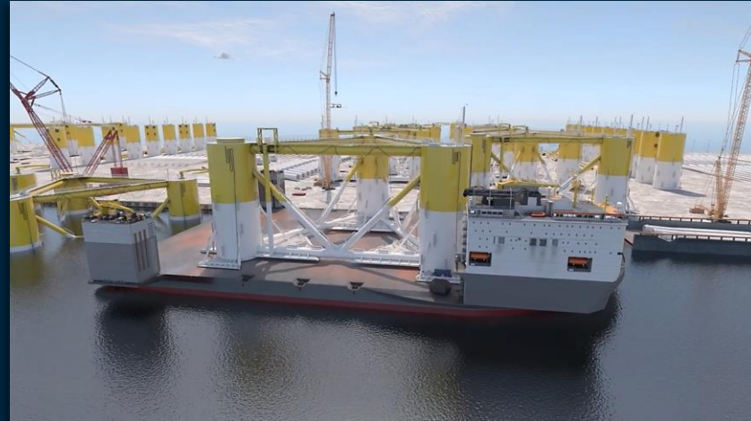
LOADOUT ONTO SEMI SUB
